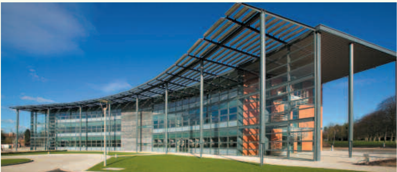
Red Kite House, the Environment Agency West Area headquarters (image courtesy of Martin Cleveland Photography for the Environment Agency).
