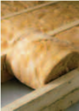
Installing insulation (image courtesy of the EST)
